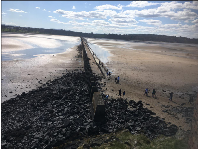
Figure 15: View of tidal walkway from Cramond Island.
